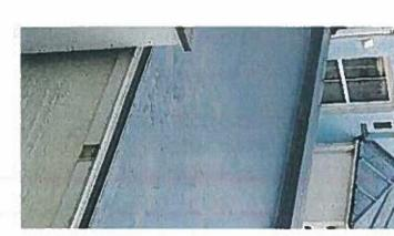
Roof – Elastomeric single ply membrane to low level flat roof
