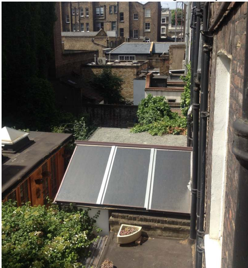
PHOTO 8: The numerous rear extensions and alterations along the rear of the terrace to the west
