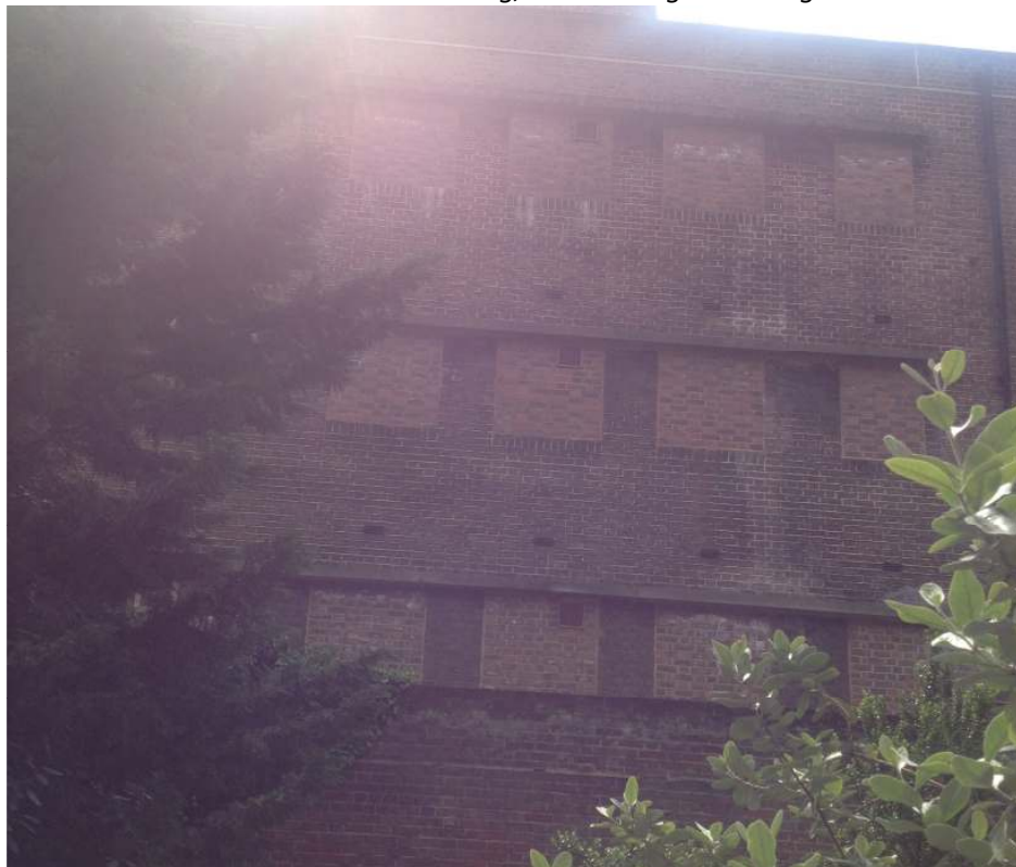
PHOTO 4: The hostel building, overlooking the rear garden
