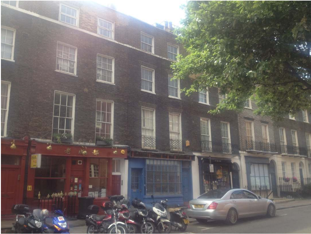
PHOTO 1: The front of the appeal terrace. The appeal property is in the centre with the blue shopfront.
