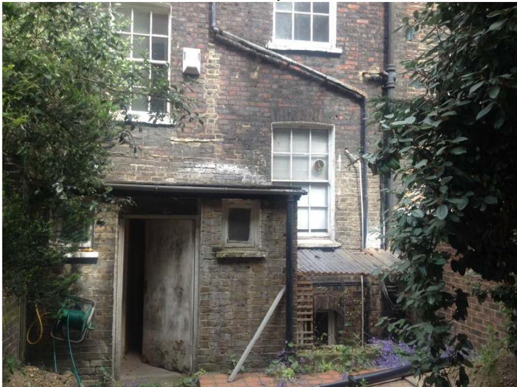
PHOTO 2: The rear of the property, with the non-original and dilapidated 20 th century rear addition to the left.
