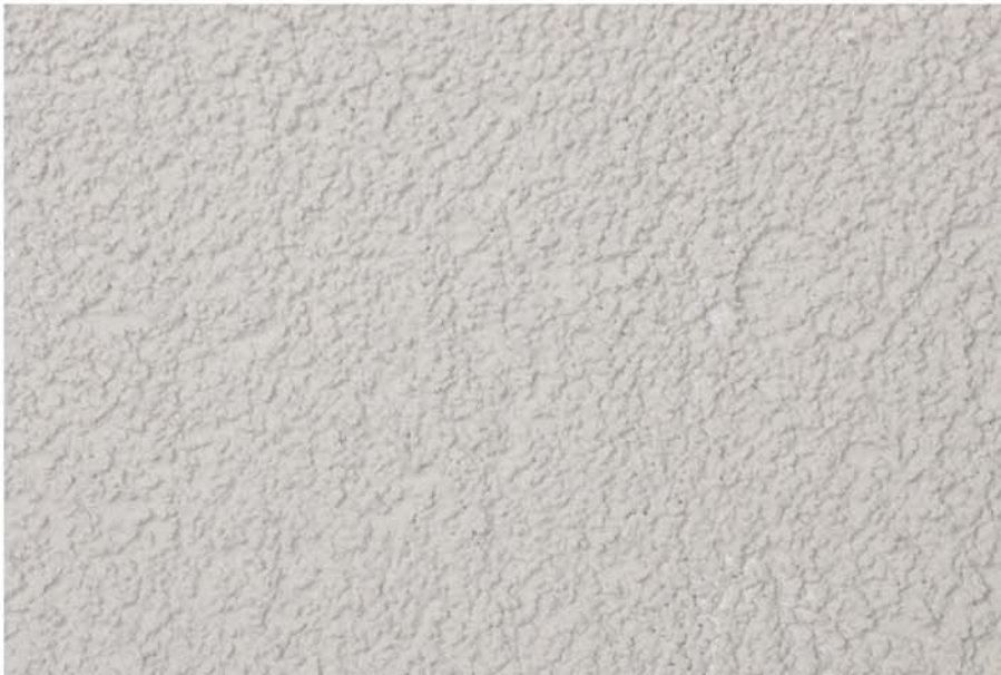
Render: West, elevation Rockwool topcoat - 1.5mm aggregate - Colour ref BC46
