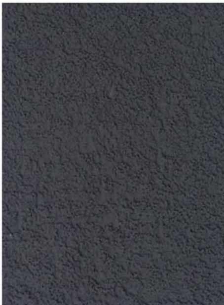
Metalwork:: North Elevation, Car Park. Rockwool Top Coat - 1.5mm aggregate - 2022
