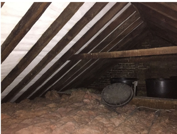
Existing roof structure to be removed
