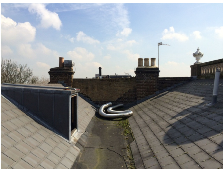
Existing roof structure to be removed
