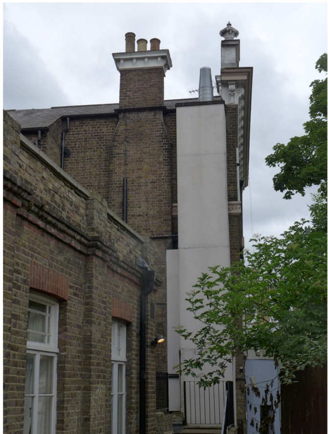
Rear elevation with restaurant extract enclosure
