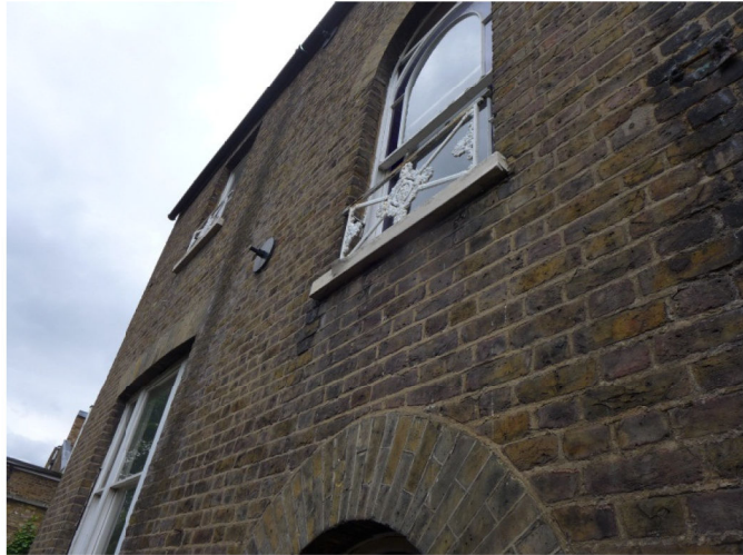
Rear brick projecting elevation with arched windows and decorative metalwork.
