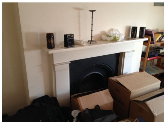
[3] First Floor front bedroom fireplace to be retained
