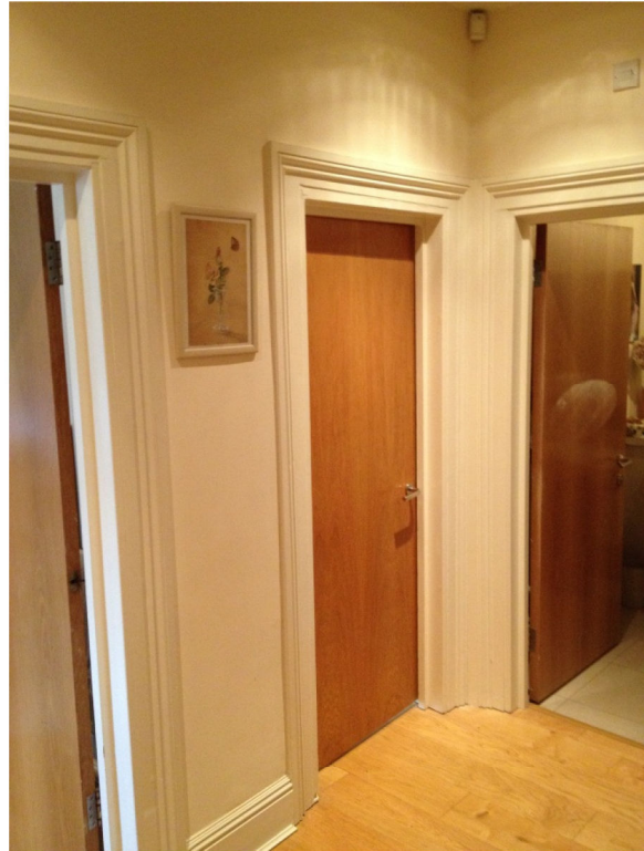
[15] Second Floor hall showing no cornice
