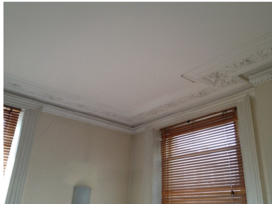
[5] First Floor living room decorative cornice
