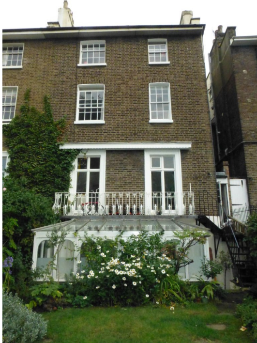
The back of 6 St Marks Crescent from the garden.
