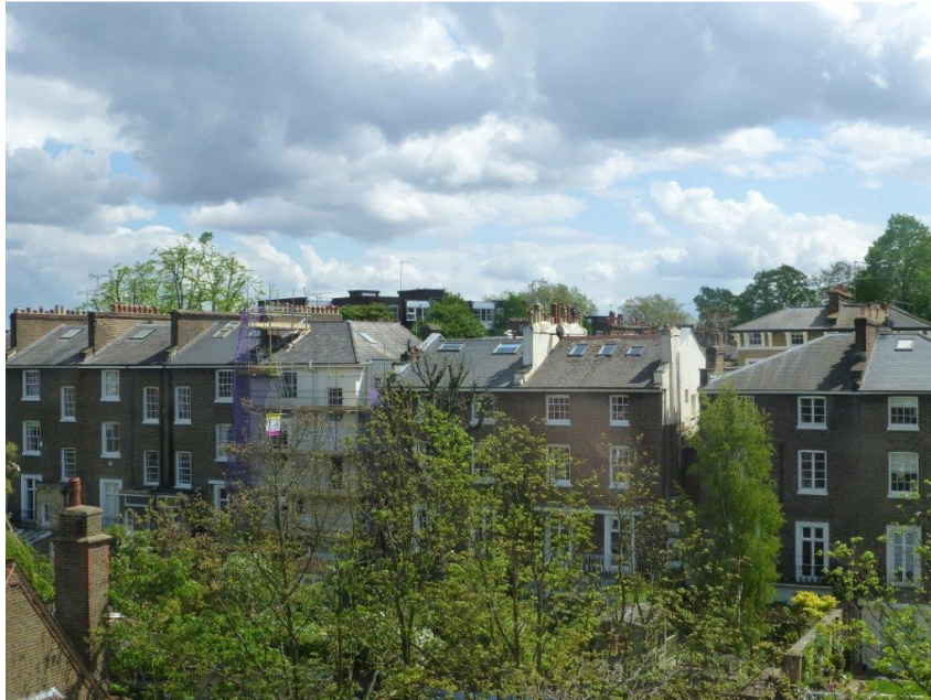
The backs of the adjoining houses in St Marks Crescent, showing the variety of existing roof lights.
