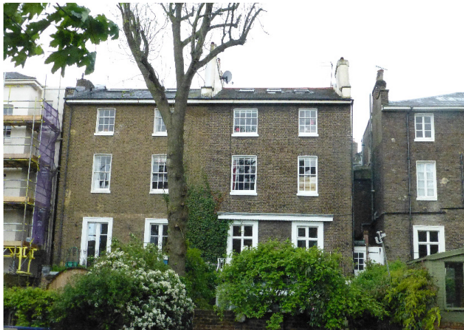
The back of 6 St Marks Crescent From the towpath. Roof lights hardly visible.
