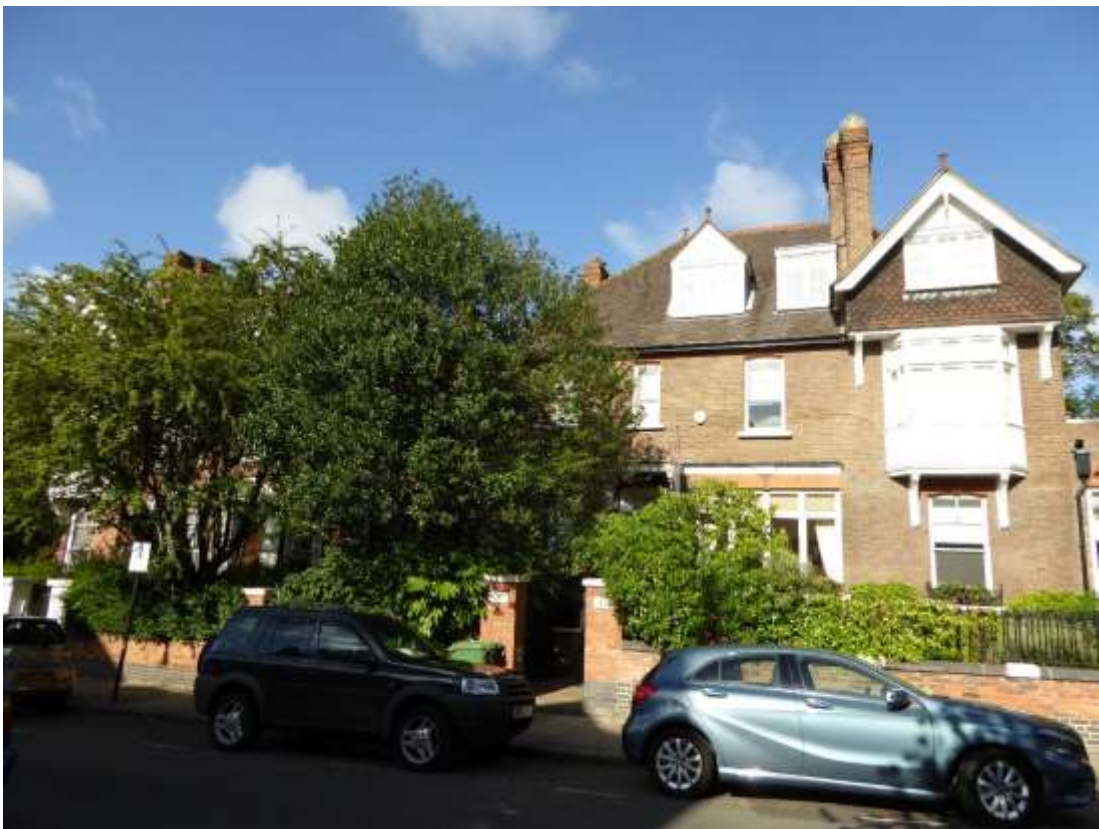
Photo 2 (RM 28.7.15) View site frontage, image taken from the east, looking west
