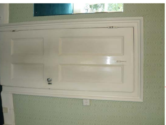
Strip and repaint timber door. Retain skirting and architrave.
