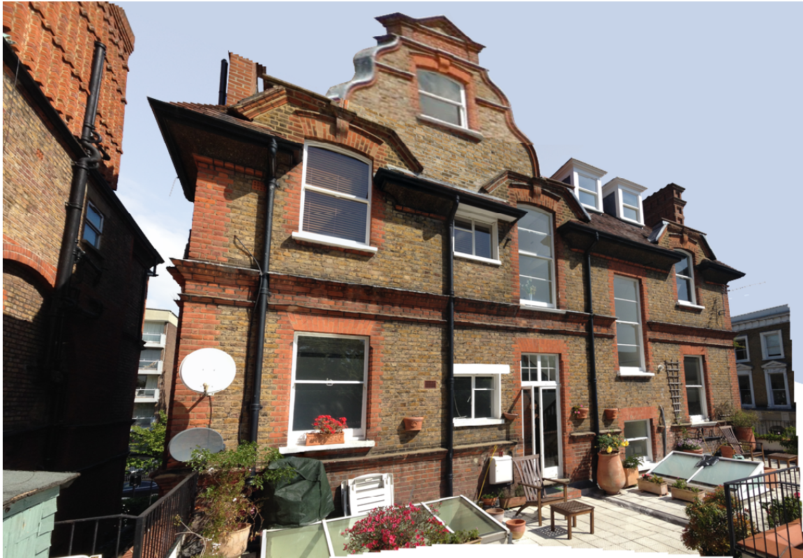
Photograph of the existing rear elevation
