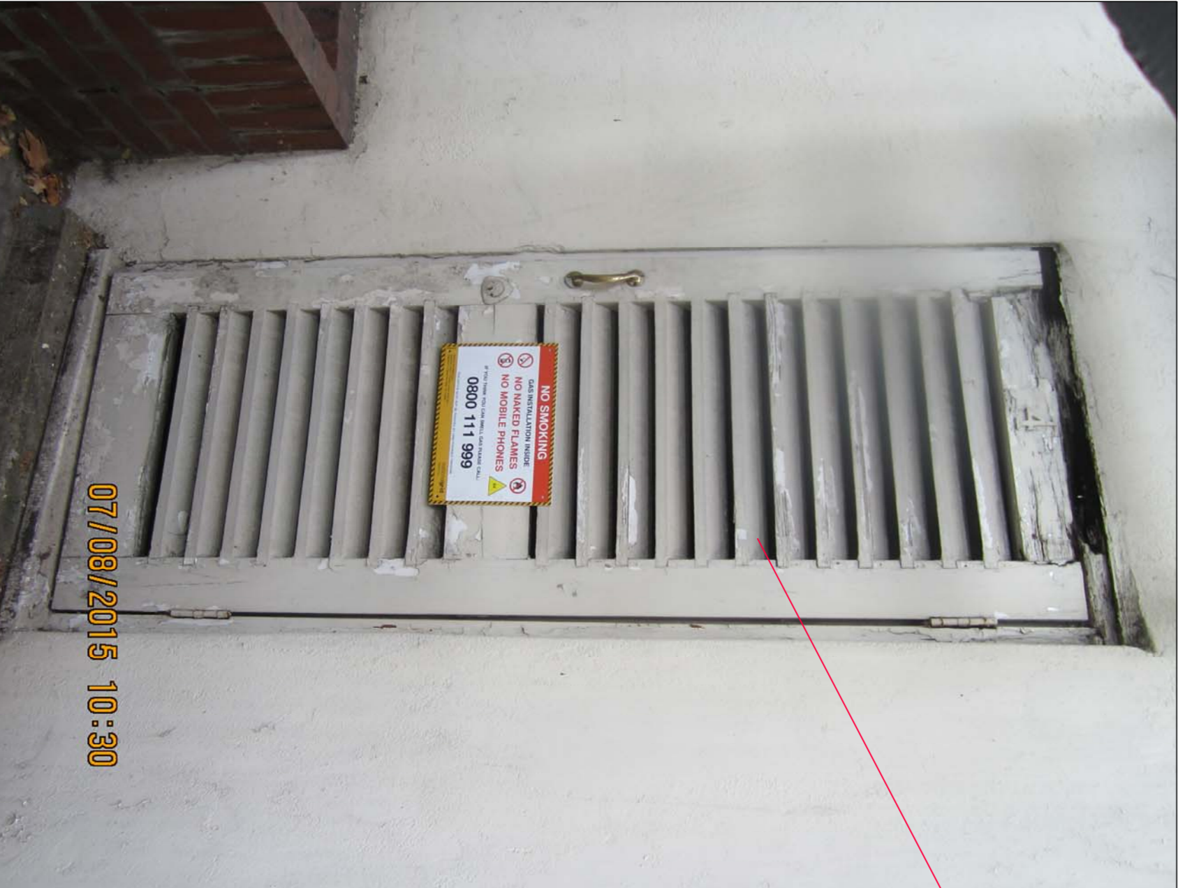
DOOR 4 EXISTING LOWERED DOORS LEADING TO VAULTED AREA BELOW MONTAGUE PLACE (N15)
