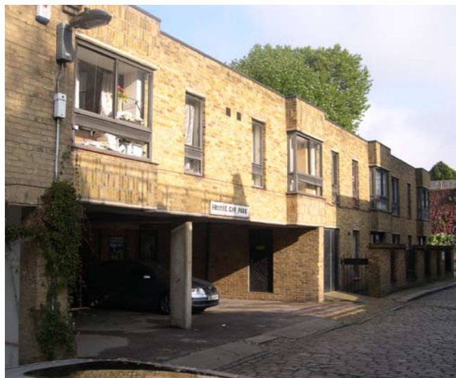
3. Ashton Court apartments on mews and undercroft
