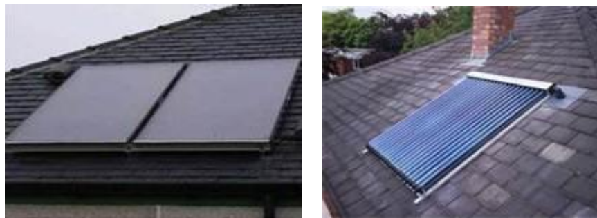
Figure A1: Flat plate and Evacuated tubes Solar Panels
