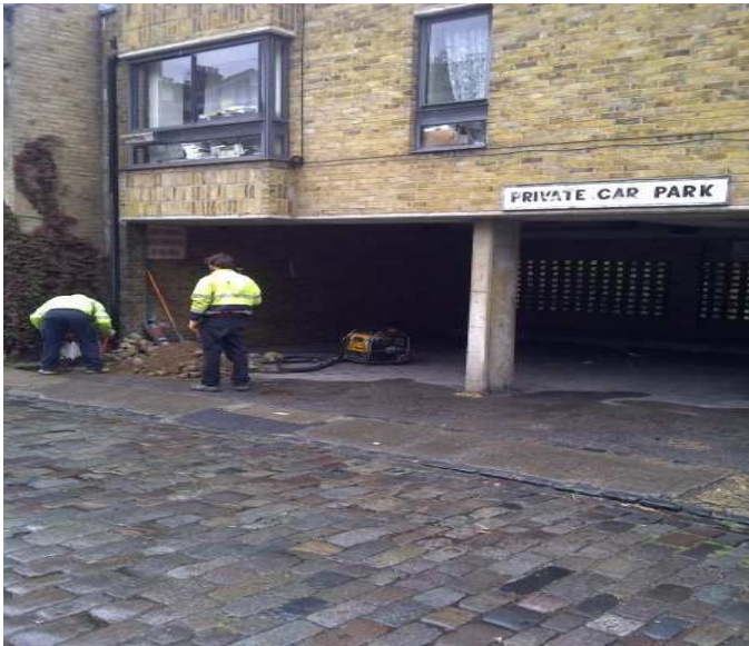
Image 5: TP2 location with party wall with 103 Camden Mews on the left
