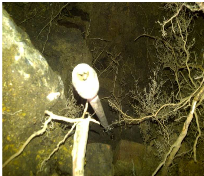
Image 4: Possible old foundations and live roots in TP1
