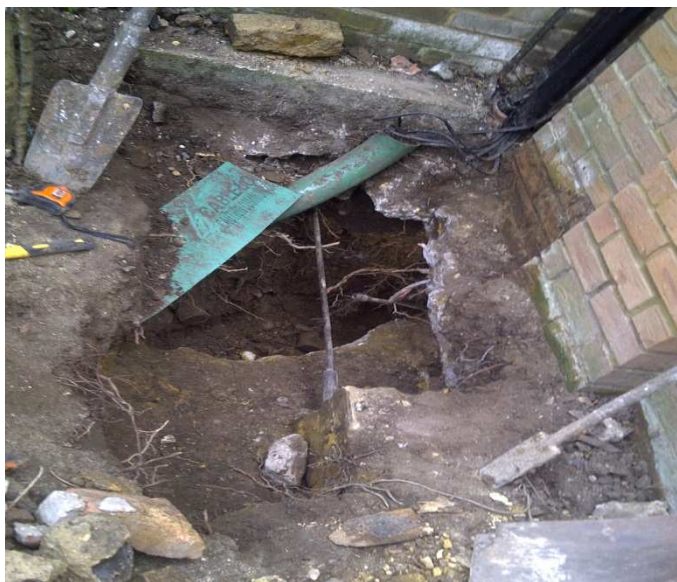
Image 3: Possible old foundations encountered in TP1
