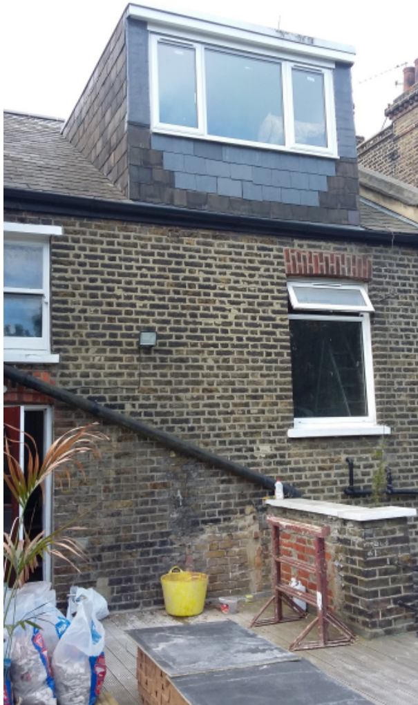
View of host building taken from existing roof terrace
