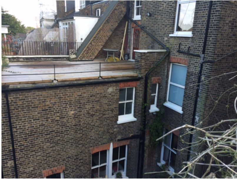
View from No. 80 towards No. 82(taken in October 2014)
