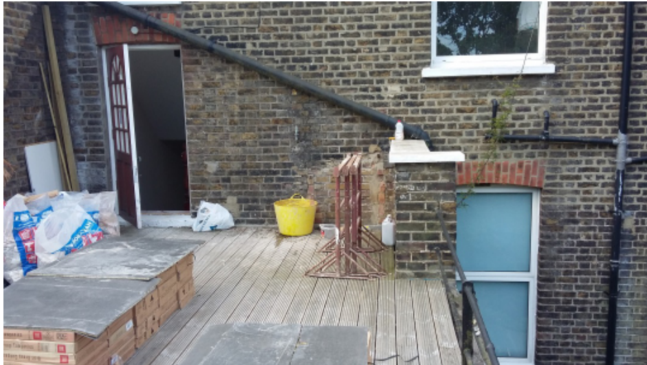
View of host building taken from existing roof terrace
