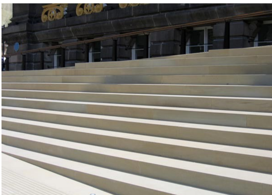
sawn york stone to form steps
