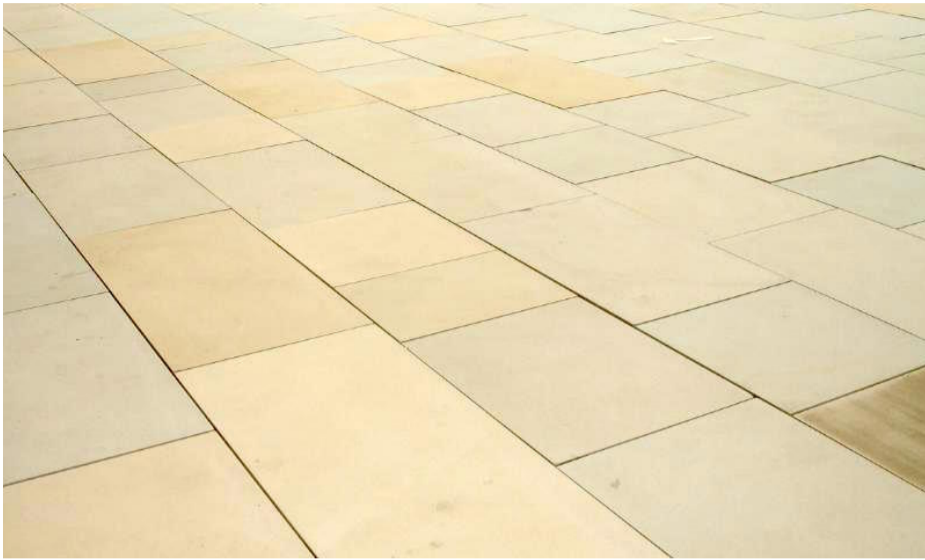
sawn york stone to front drive
