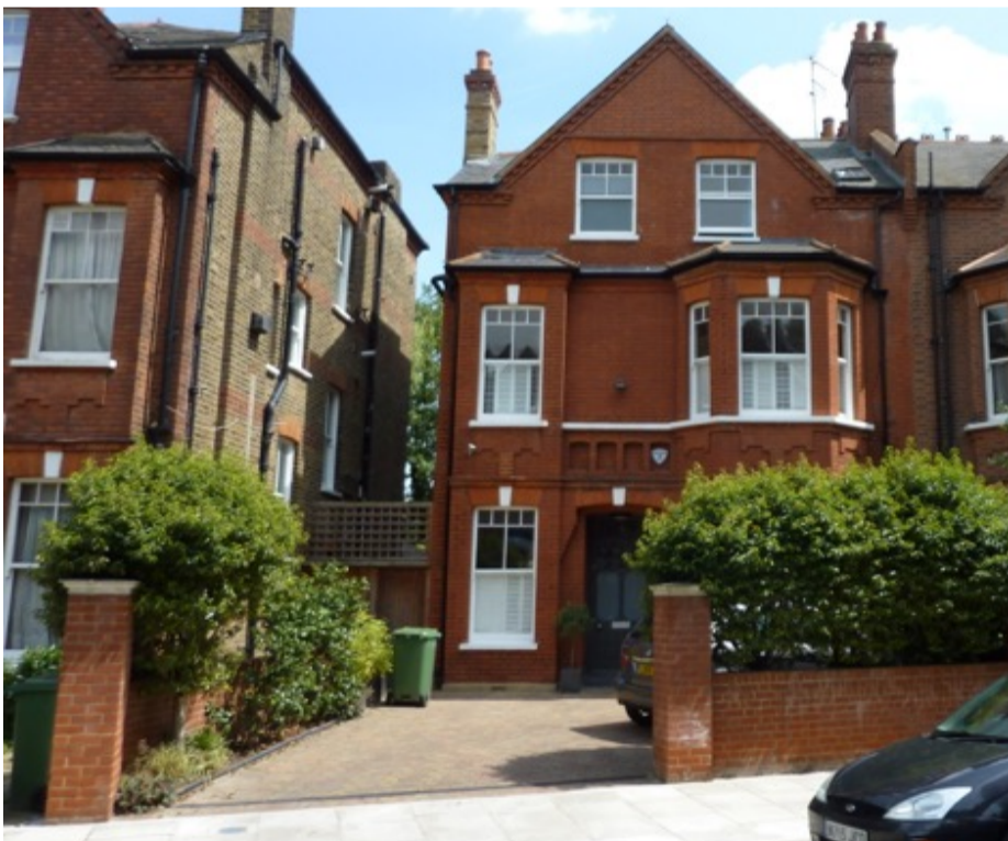
the front facade (prior to refurbishment works)
