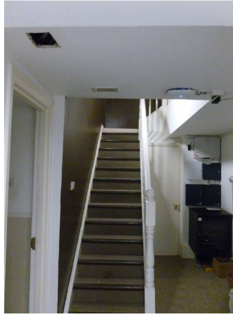
Image of existing internal basement stair.
