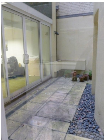
EXISTING BASEMENT PATIO AREA
