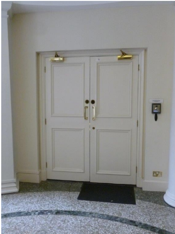
PICTURE OF EXISTING OFFICE SUITE ENTRANCE DOORS SOUTH SIDE THIRD FLOOR.
