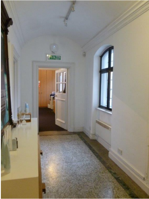
GRANOLITHIC FLOOR NORTH SIDE INNER LOBBY.
