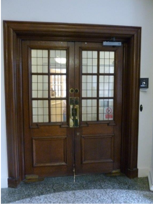
EXISTING LOBBY ENTRANCE DOOR NORTH SIDE
