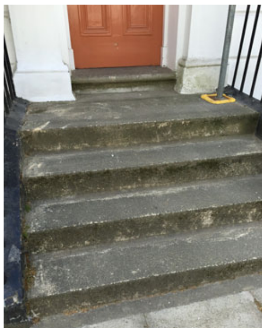
View showing concrete replacement steps to front door.
