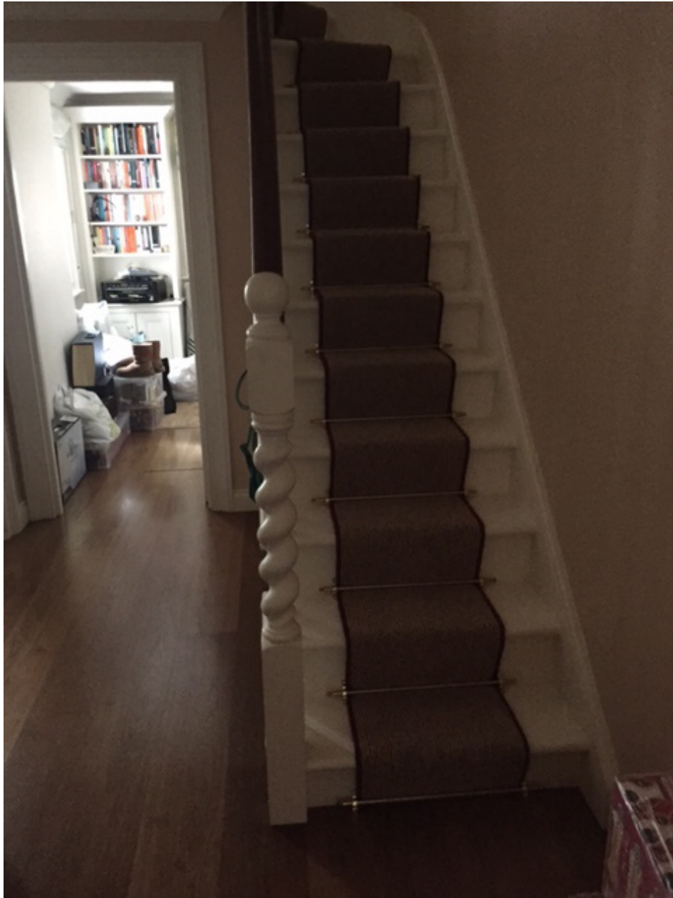
Image of next door neighbours stair, supporting opinion that current winder-stair arrangement is not original
