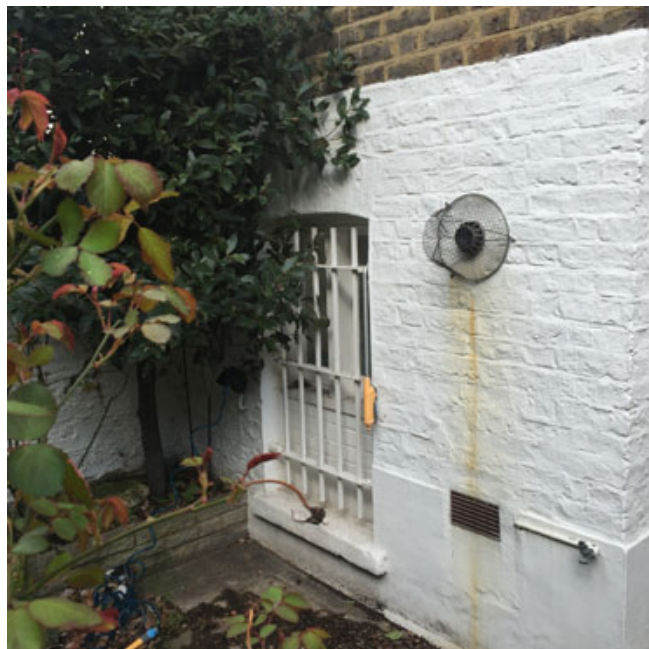
View of base of closet wing showing painted brick modern window and brick infill to original opening.
