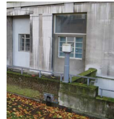
Type W - refurbished and retained in location
