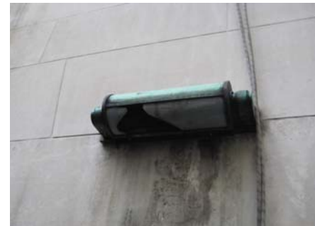
Type U - refurbished and relocated into new courtyard
