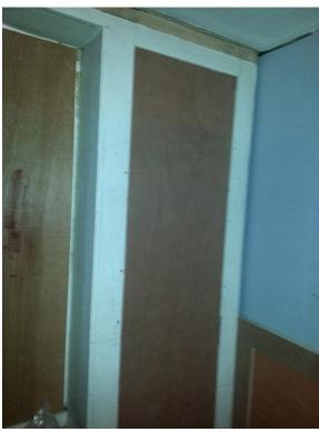
2. Where building entirely new panels on top floor we would use ply with soft wood stiles and mouldings to get the best finish as shown in sample below.
