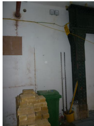
Wall viewed from unit G27 looking towards unit G25
