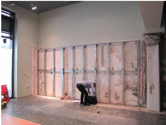
Wall viewed from unit G25 looking towards unit G27
