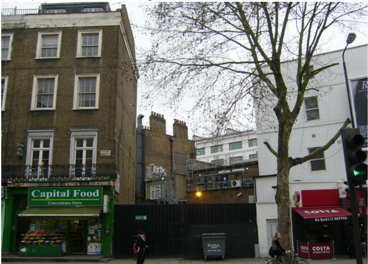
(Photo 2) Rear of terraces at Hurdwick Place and Eversholt Street
