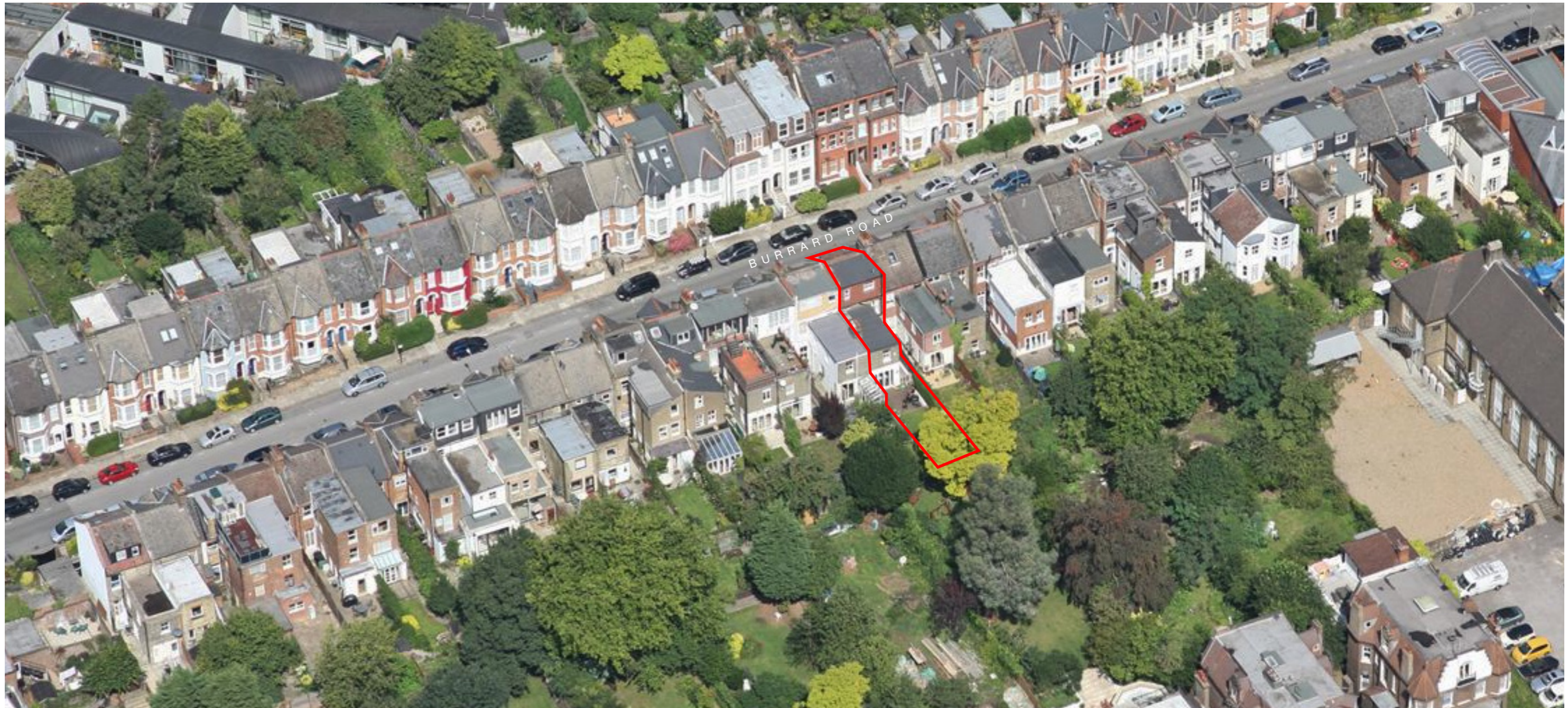
02. aerial view north
