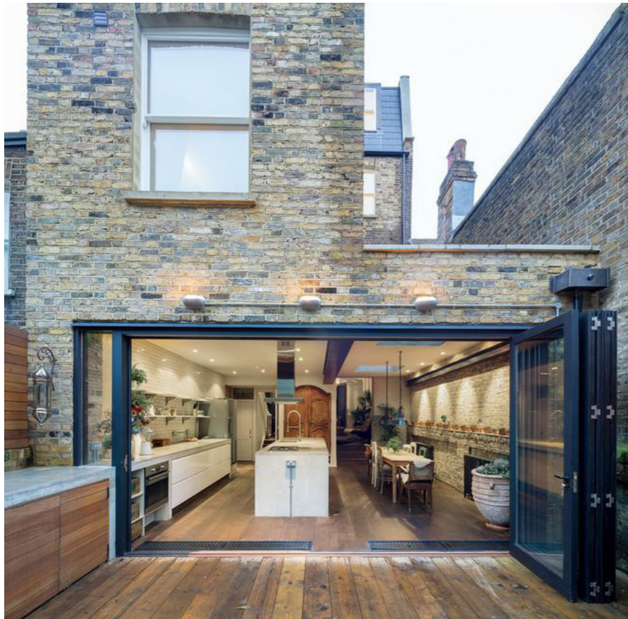
01. high quality brickwork and glazed bi-folding doors
