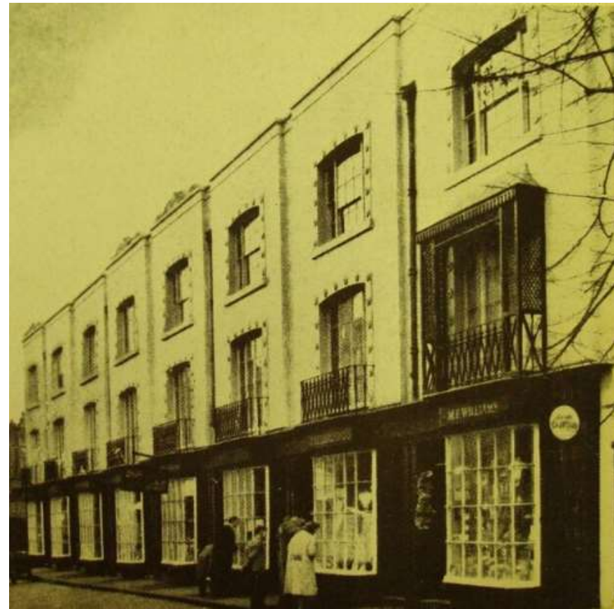
Figure 10: 1-7 Woburn Walk, Post-1961 & Restoration
