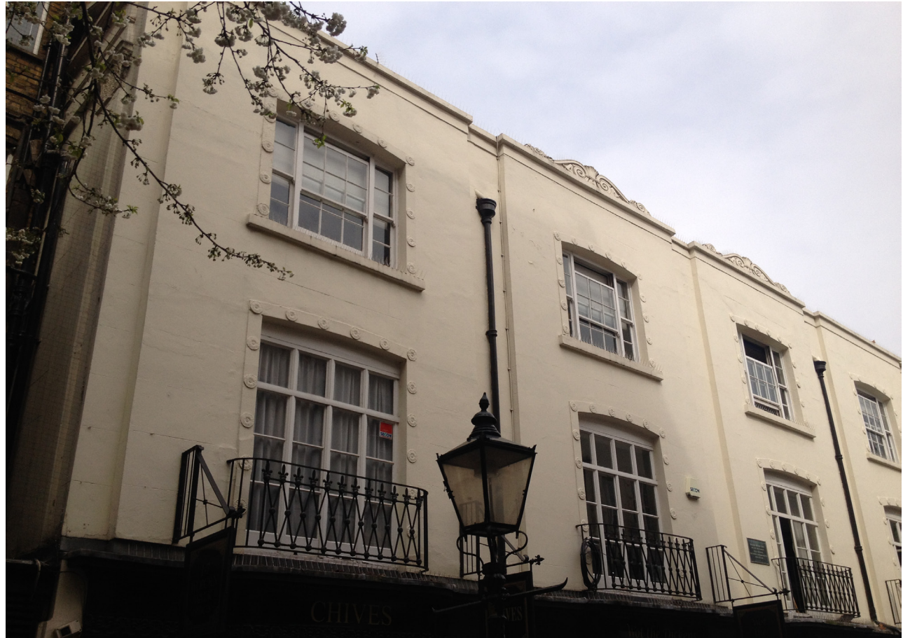
Front façade showing the first and second floor windows facing Woburn Walk. The plaque denotes the historic significance of its famous former resident.
