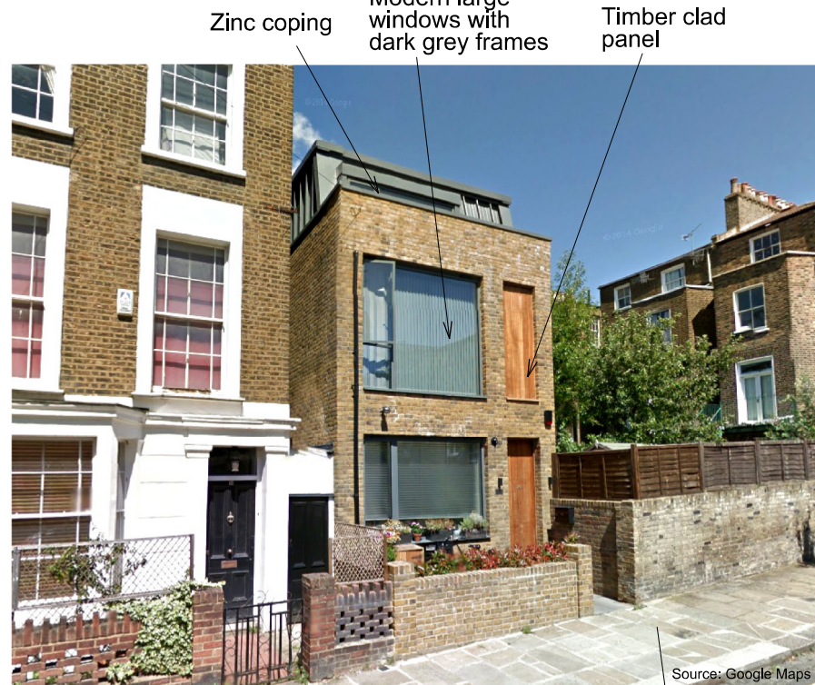
14a St Pauls Crescent (Example of large dark grey powder coated windows and use of timber on front elevation)
