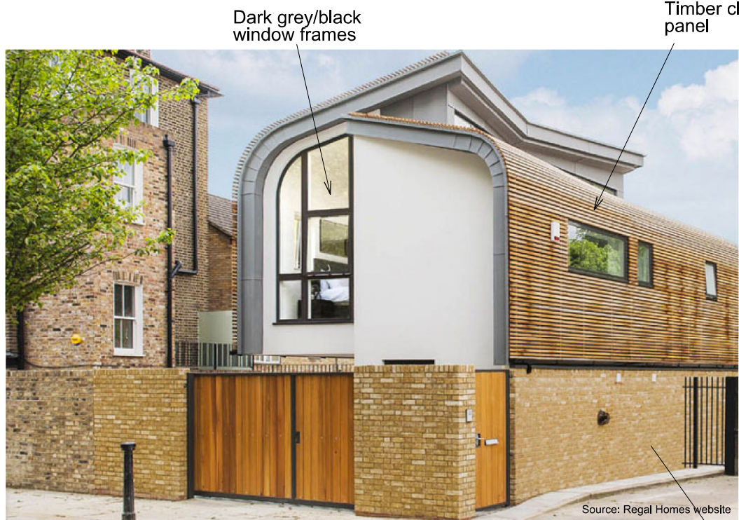
36a St Pauls Crescent (Example of dark grey / black metal frame windows, render wall and timber cladding)
