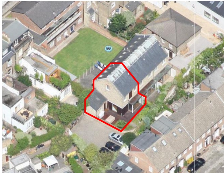
Figure 2-1 View of the Existing building at 41A Ivy Road
