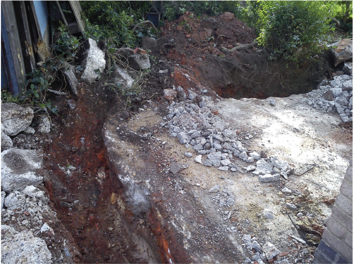
Photo 5 – TP302: Edge of building foundations
