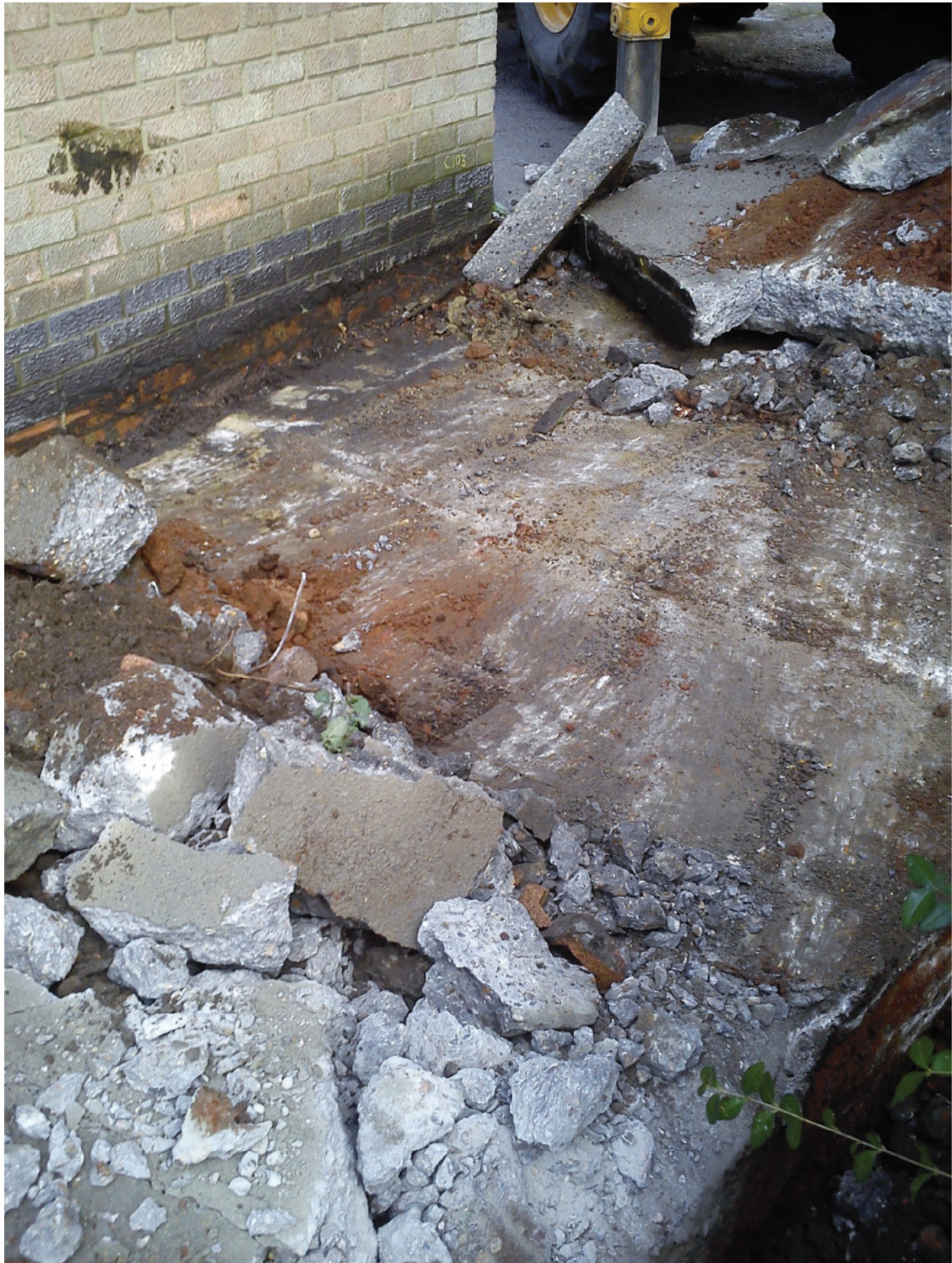
Photo 2 – TP302: Building Foundations
