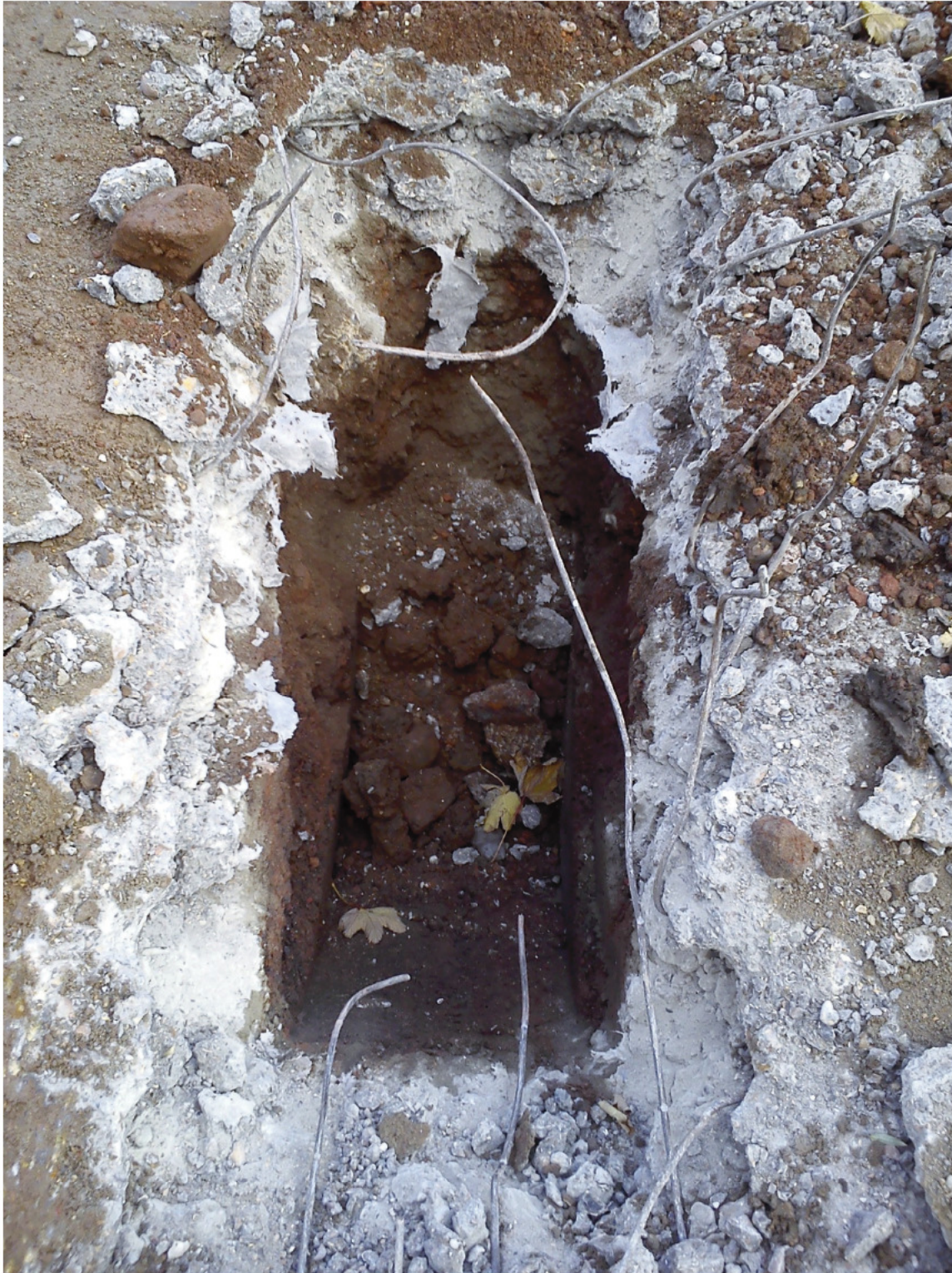
Photo 4 – TP304: No brick wall encountered
