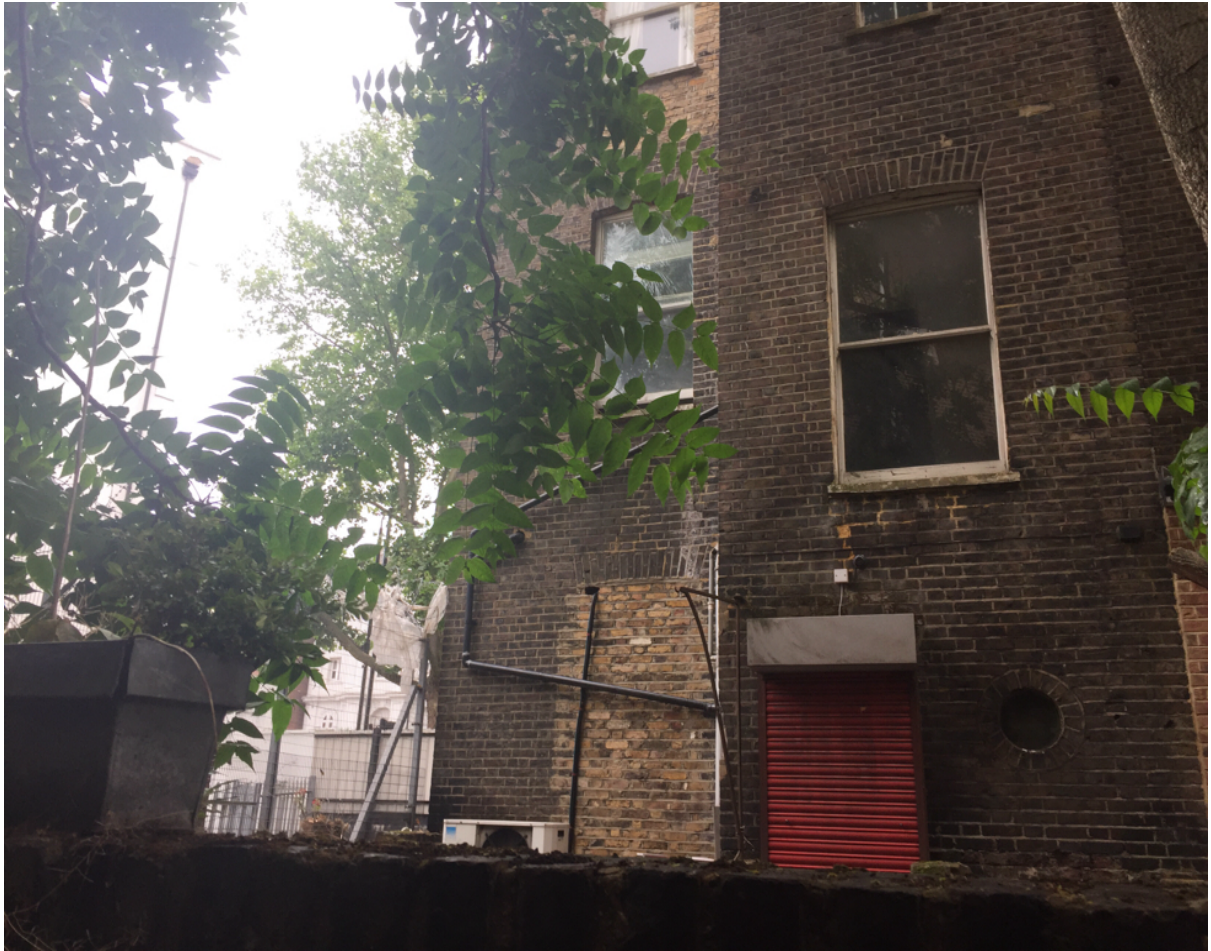
(Photo 5)Rear looking east
