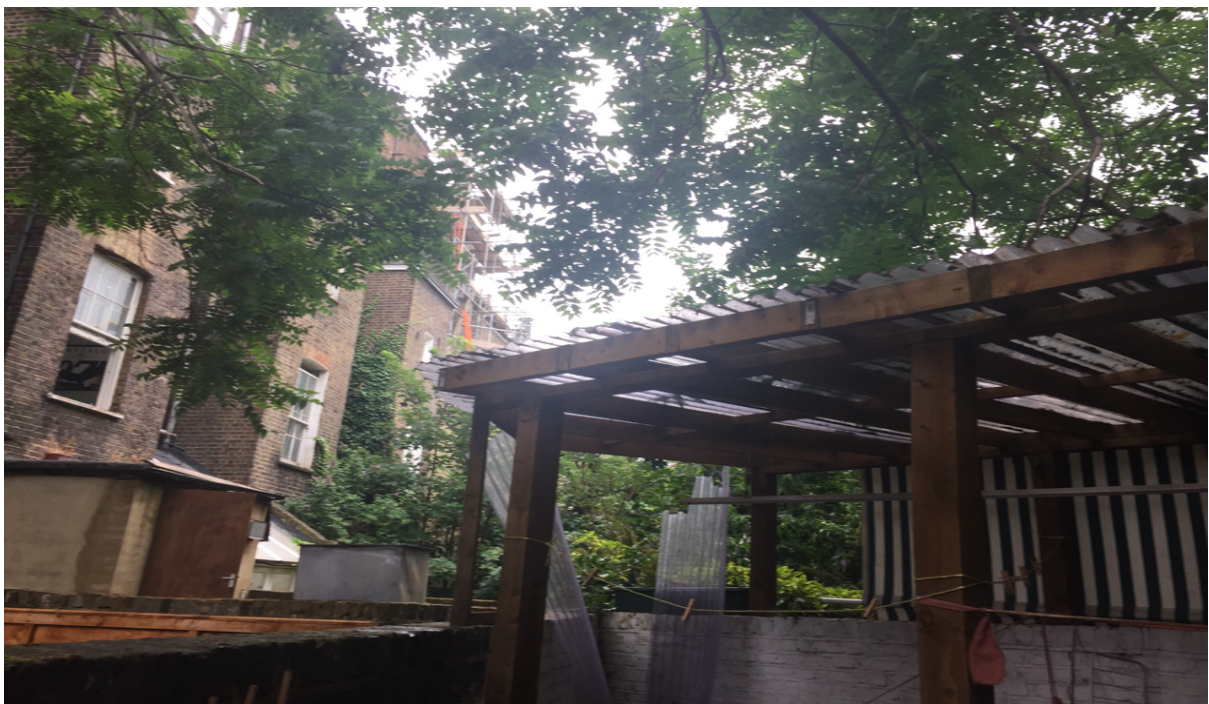
(Photo 4) Existing rear extension
