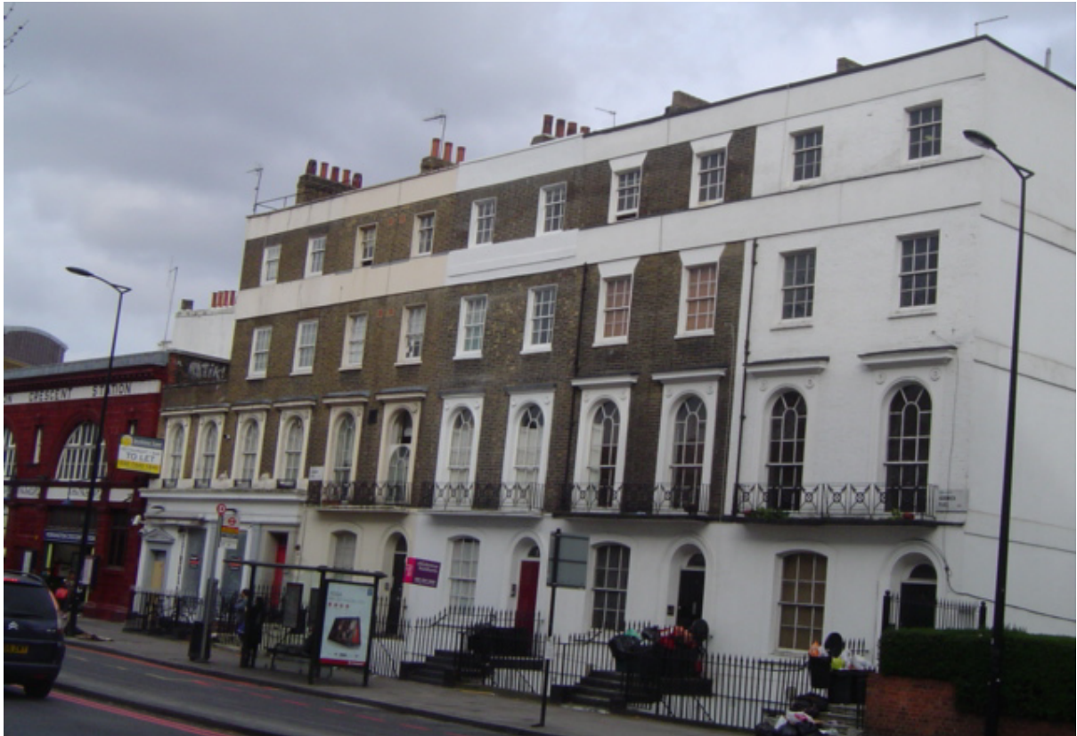
(Photo 1) Front of the terrace area looking east
