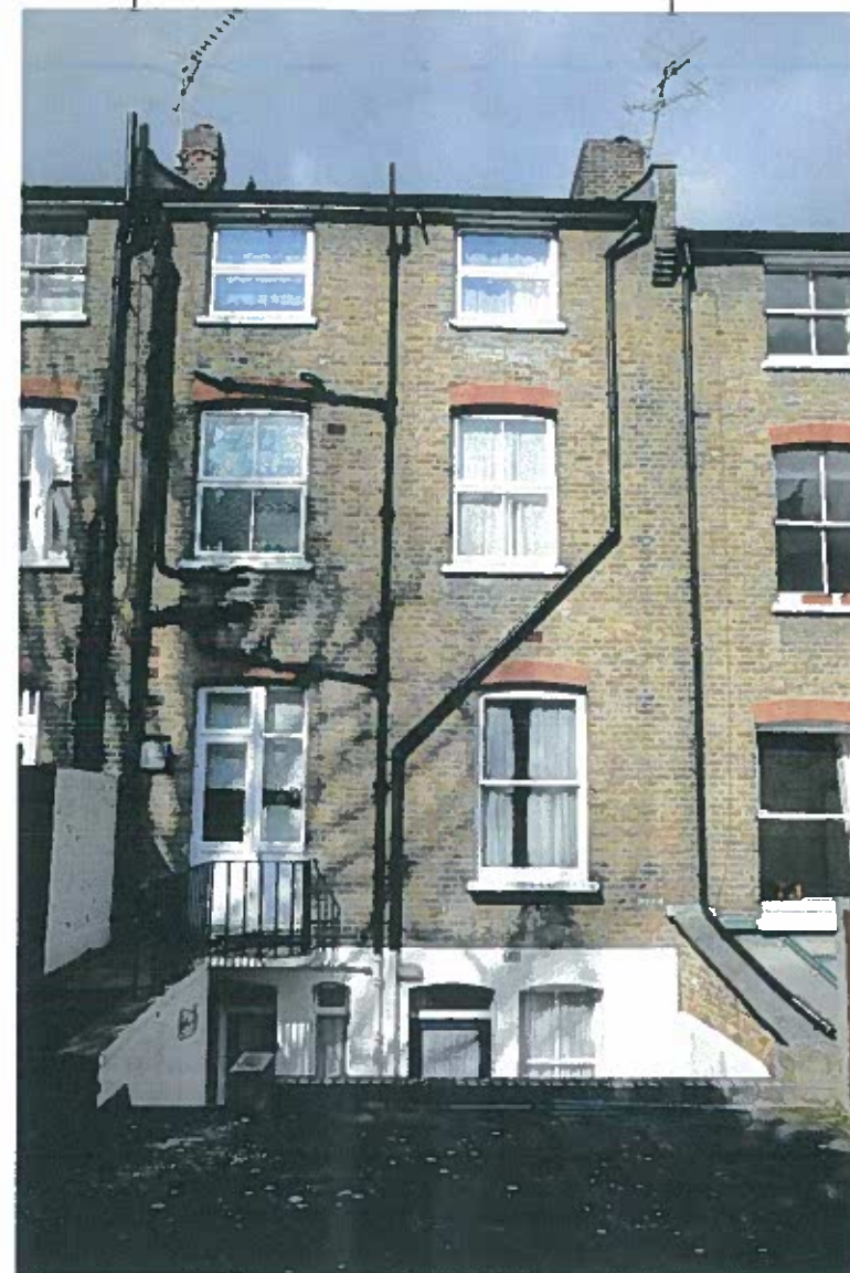
18 DENNING ROAD EXISTING VIEW FROM GARDEN.
