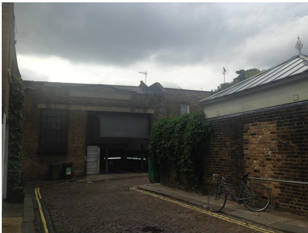
Figure 15: View of site from Leverton Street, the rear garden of the Pineapple Pub on the right.
