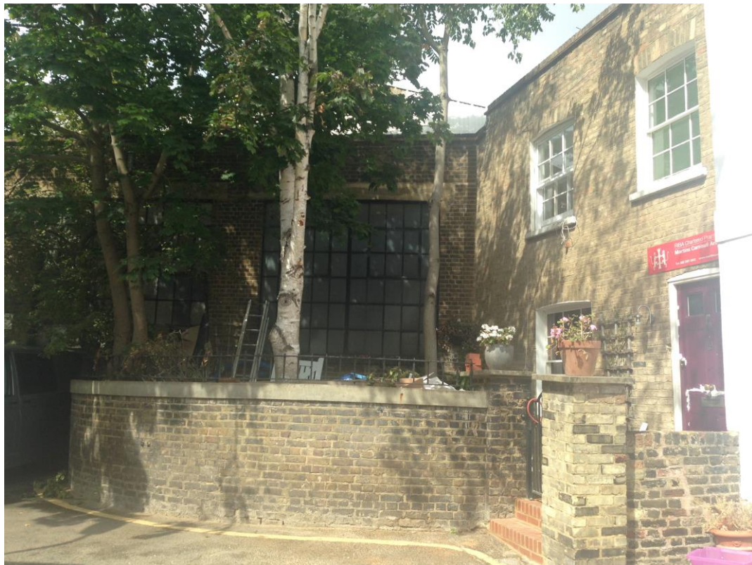
Figure 14: View of Site from Fortess Grove, No 1 Fortess Grove to the right.
