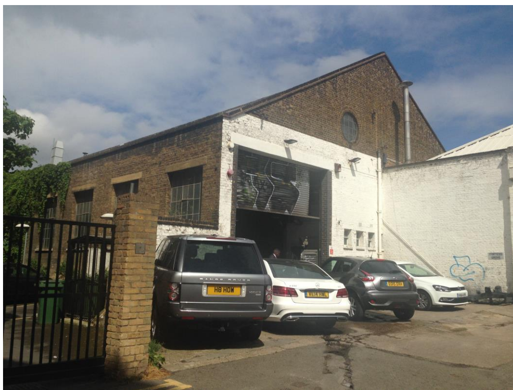
Figure 8: Warehouse at Fortess Grove.
