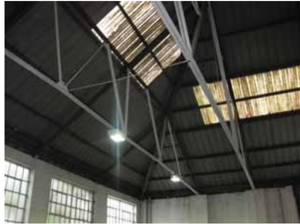
Internal of the small warehouse. Steel beam supporting roof rafters above large opening (left) and roof trusses (right).
