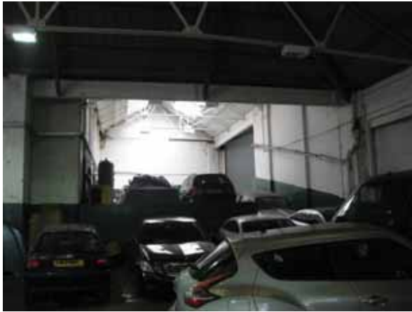
Internal of the small warehouse. Steel beam supporting roof rafters above large opening (left) and roof trusses (right).
