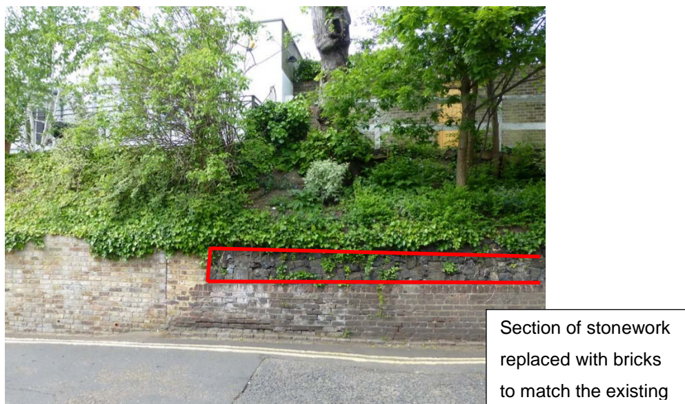
Photograph #9: showing existing retaining structure to be replaced with bricks matching the existing (only the dark stone above the existing wall is being replaced)
