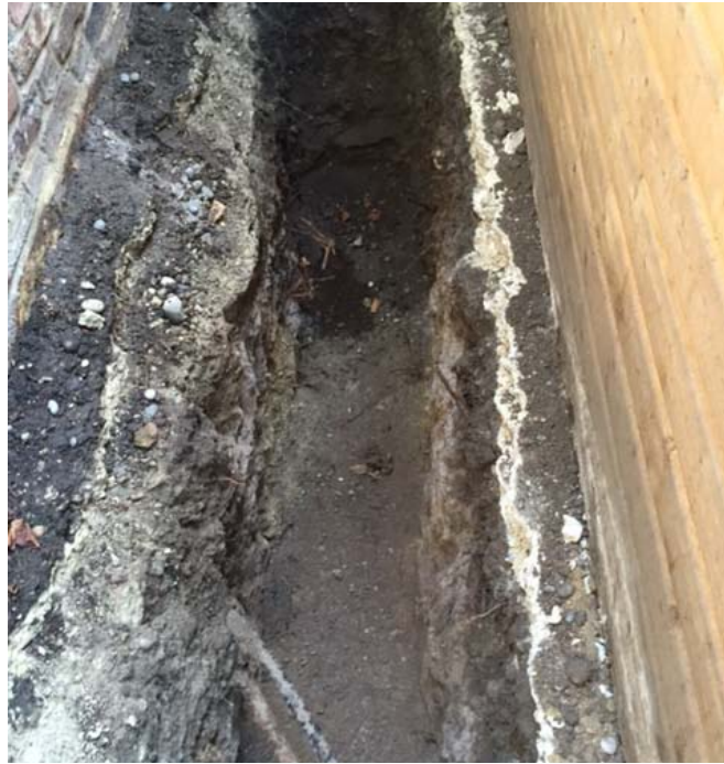
Photograph #4 – showing the second stage of the excavation to a depth of 700mm with no roots encountered
