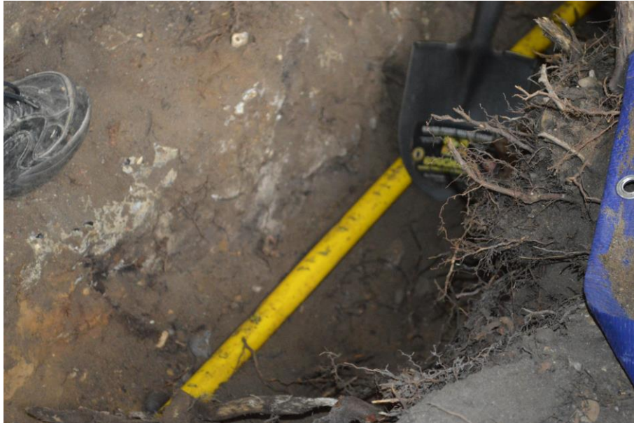
Photograph 4 Gas pipe running alongside the garage wall.
