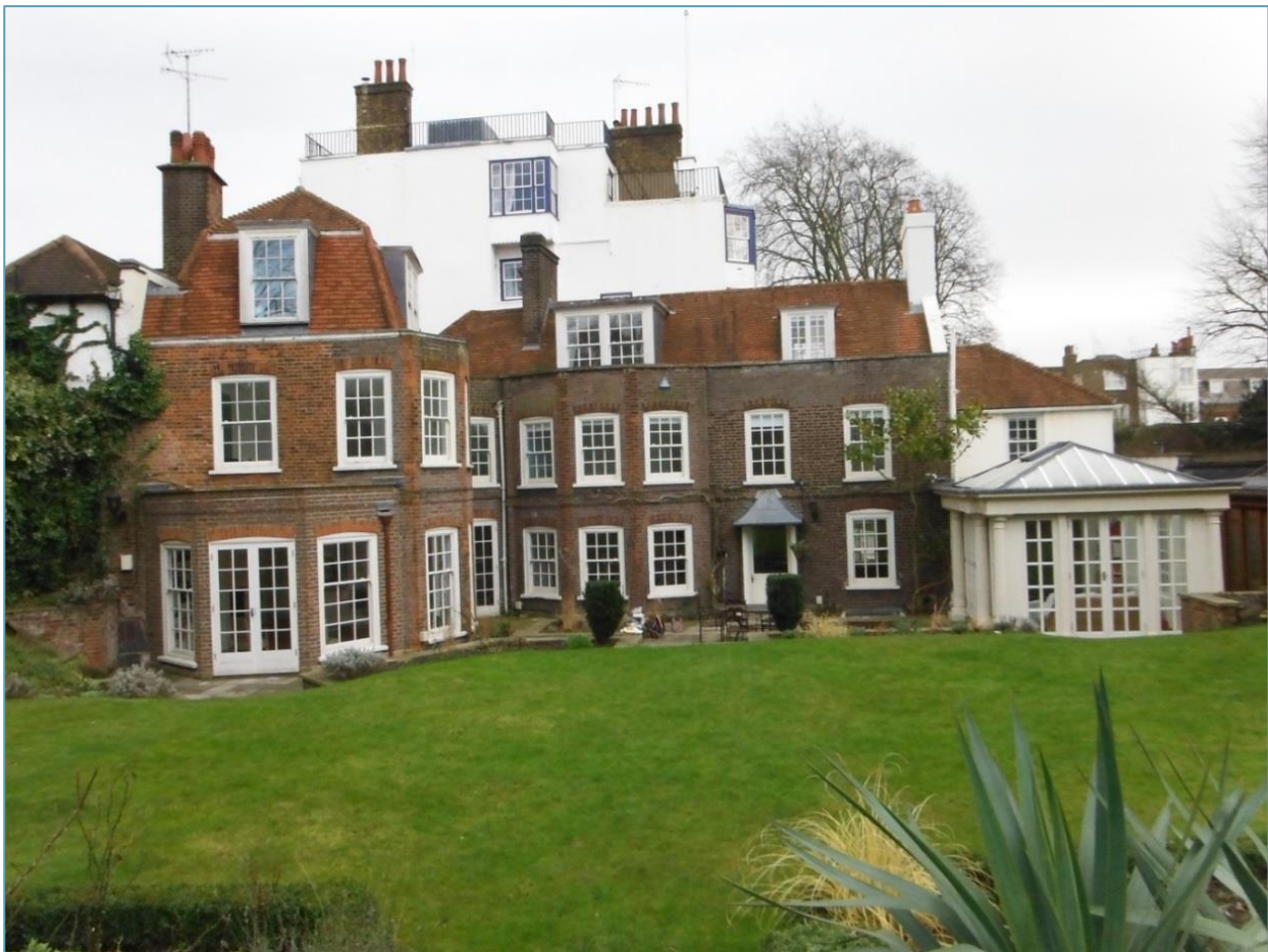
Photograph 3.2: Grove Lodge: rear view – from within garden: basement location
