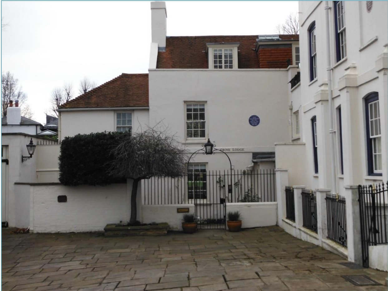
Photograph 3.1: Grove Lodge: front view – from Admiral's Walk. Admiral's House on the right
