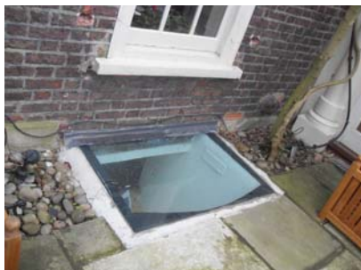
Existing lightwell to the rear
