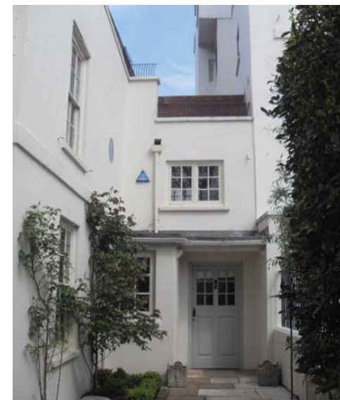
Fig 6: Front Entrance view from forecourt
