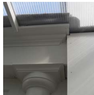
Southern extension, interior
