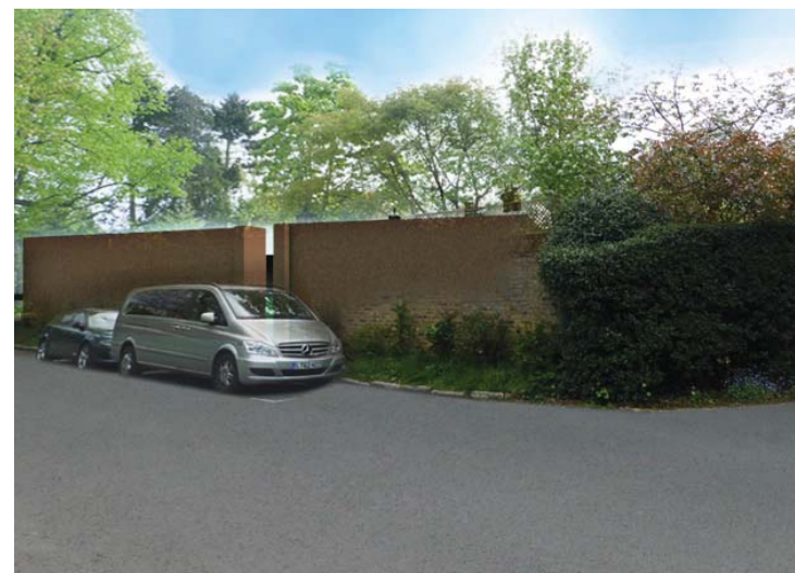
Fig 34: Street level view from Lower Terrace
