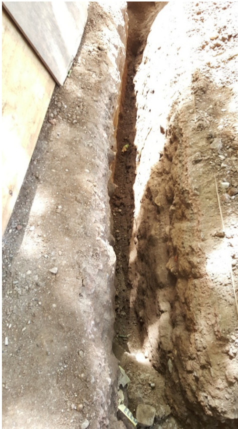
Photograph 3 and 4 (29-06-2015) 2 Views into the trench showing the densely compacted inert fill material and absence of roots.
