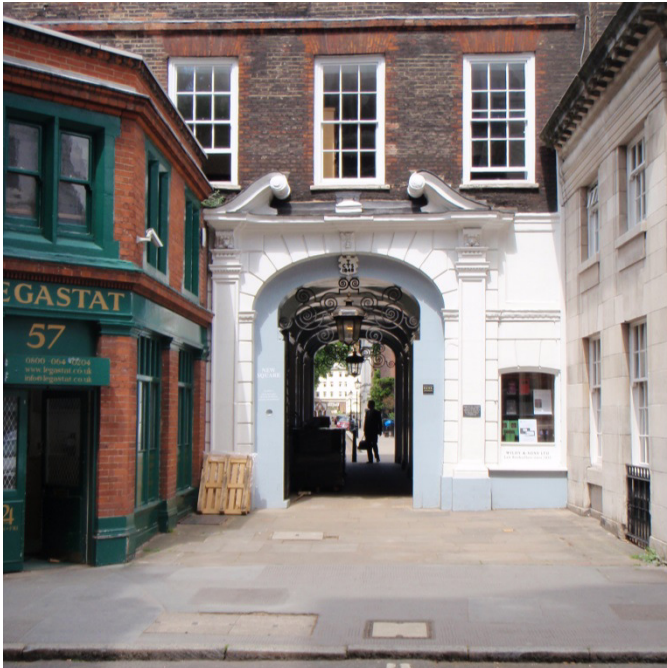
Figure 2.4: Main Pedestrian Access from Carey Street
