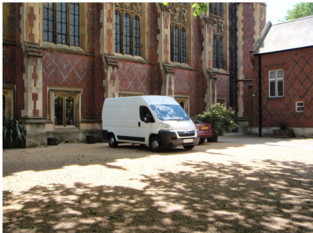
Figure 2.7: Disabled Parking by the Library
