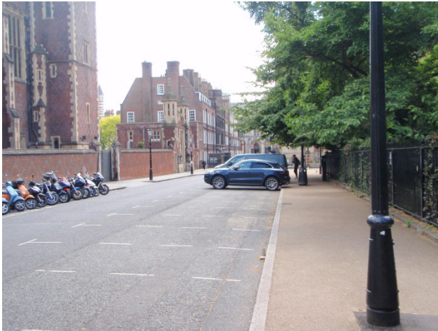
Figure 2.11: Existing Footways on Newmans Row
