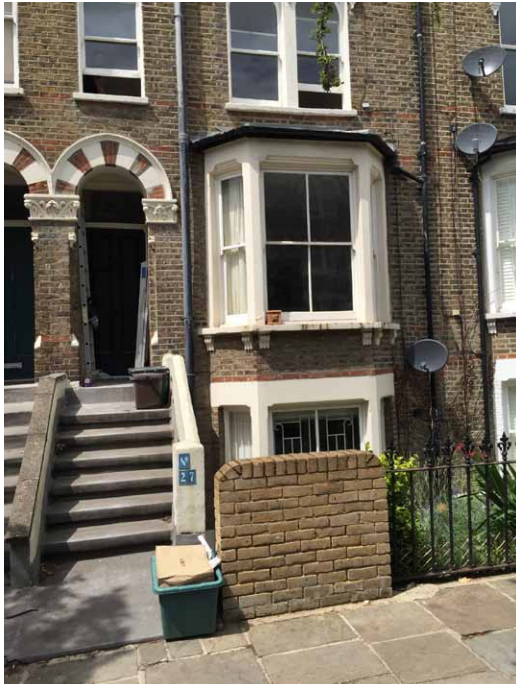
Right; Front elevation and main entrance to 27 Lowfield Road
