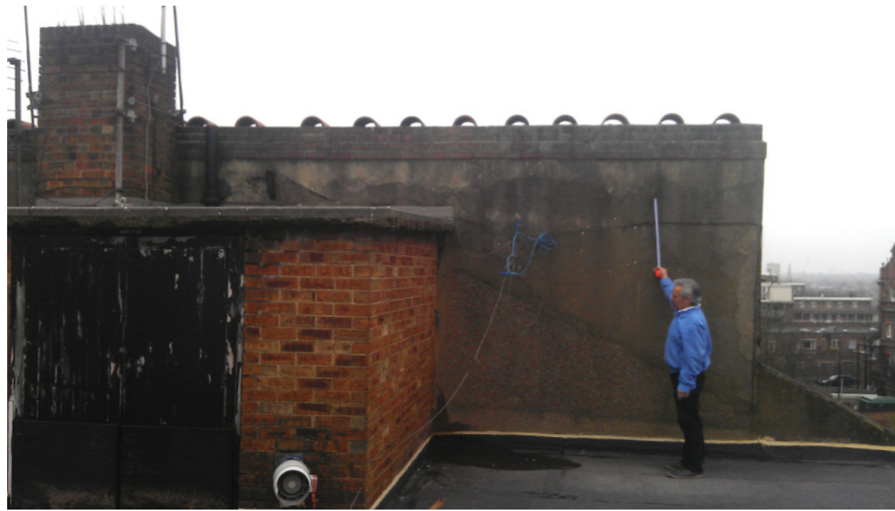
Existing Flat Roof & Party Wall
