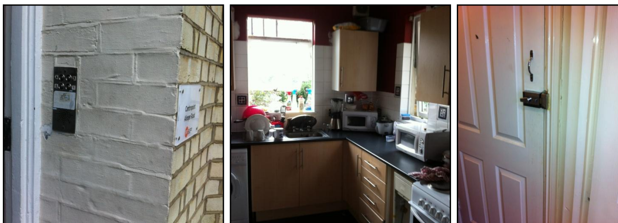
12 Ainger Road - Doorbells to individual flats on lower ground, ground, first and second floor level (Left); Example of an individual kitchen within each flat (Middle); and Example of a locked front door to each flat (Right)
