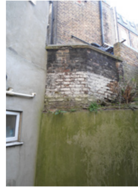
Basement patio in number 121
