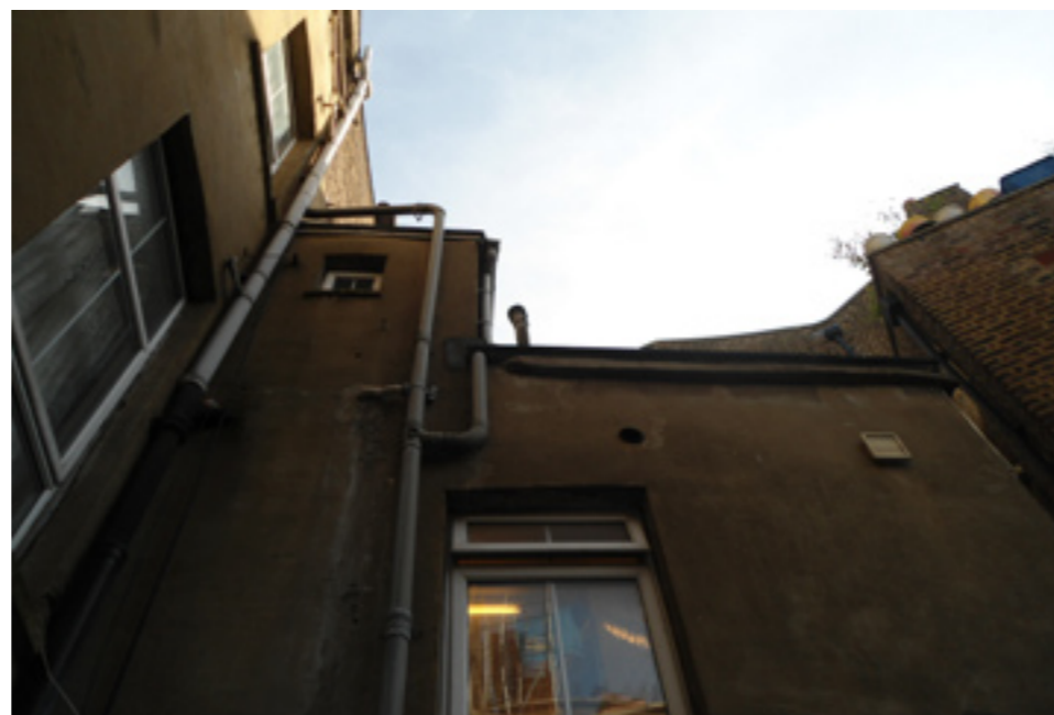
Volume sticking out of the main rear facade in number 121
