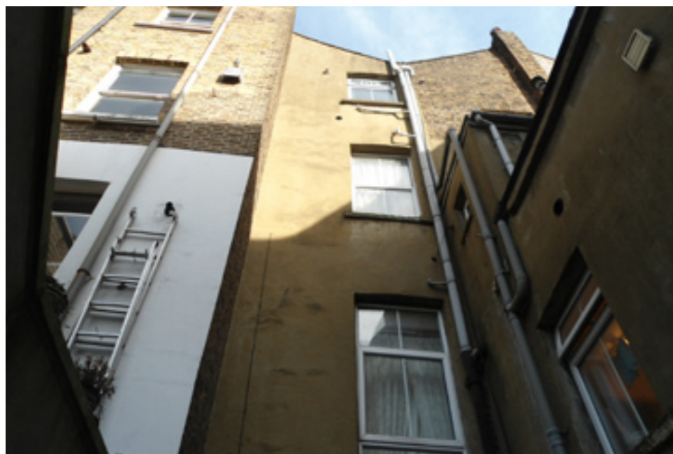
Rear facade in number 121
