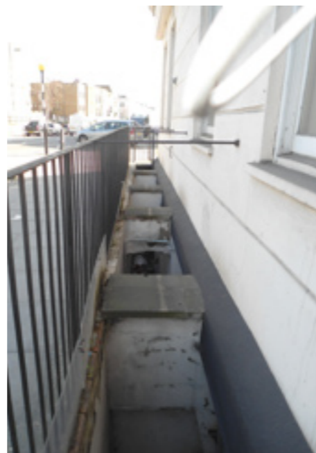
Basement access in number 117 malden road
