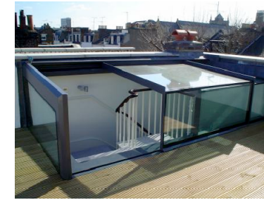
2 Lightweight structure to roof access. Glazing to be low g value to avoid solar heat gain. Image for reference only.
