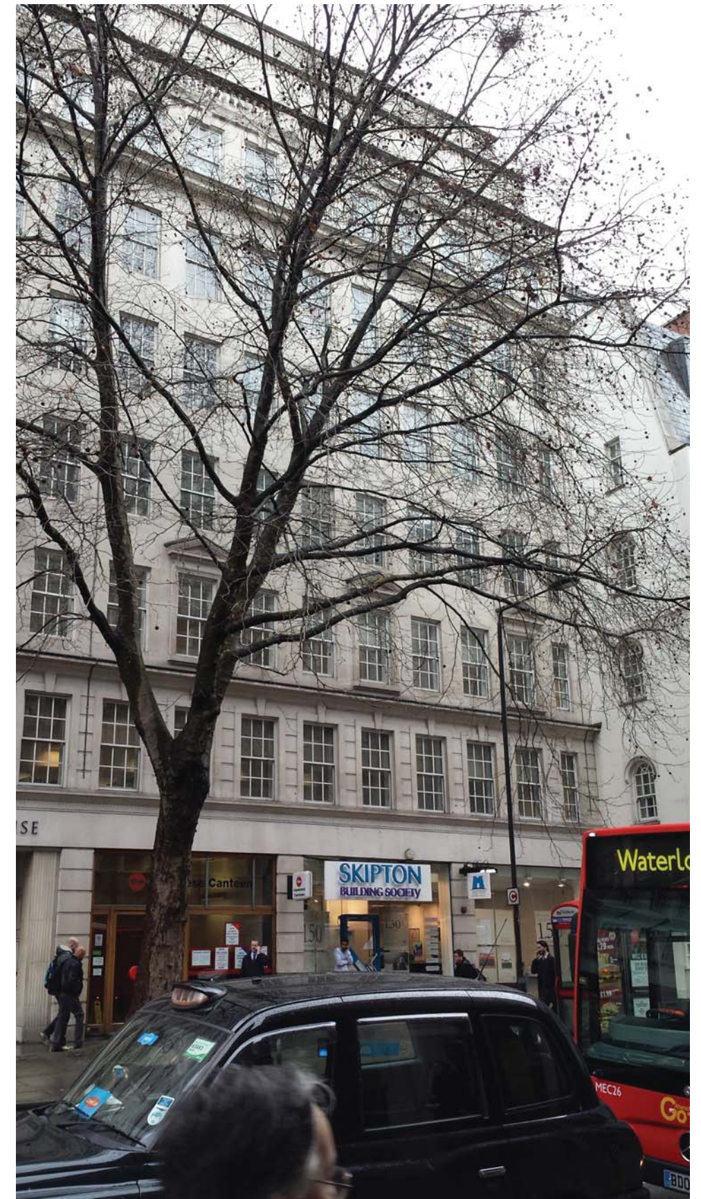
TEMPLAR HOUSE CURRENT FACADE TOWARDS HIGH HOLBORN
