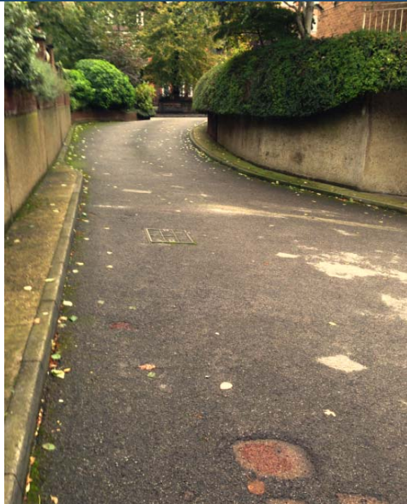
Figure 41 Avenue Road runs down into garage areas
