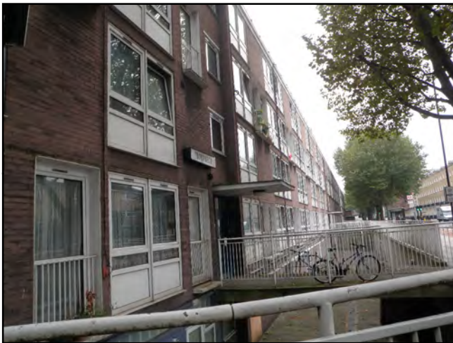
Photograph 3: The Troutbeck Overbuilds (Building 3) was also assessed to have negligible potential to support roosting bats.
