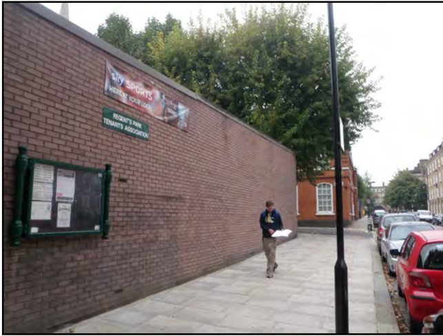
Photograph 1: Building 1 (including the Dick Collins Community Hall) was assessed as having negligible potential to support roosting bats.
