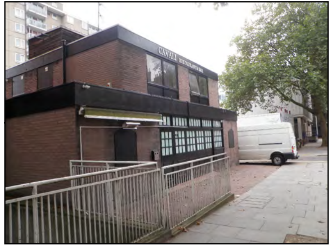
Photograph 2: No features suitable for roosting bats were identified on Building 2 (Cavalli Restaurant and Bar).
