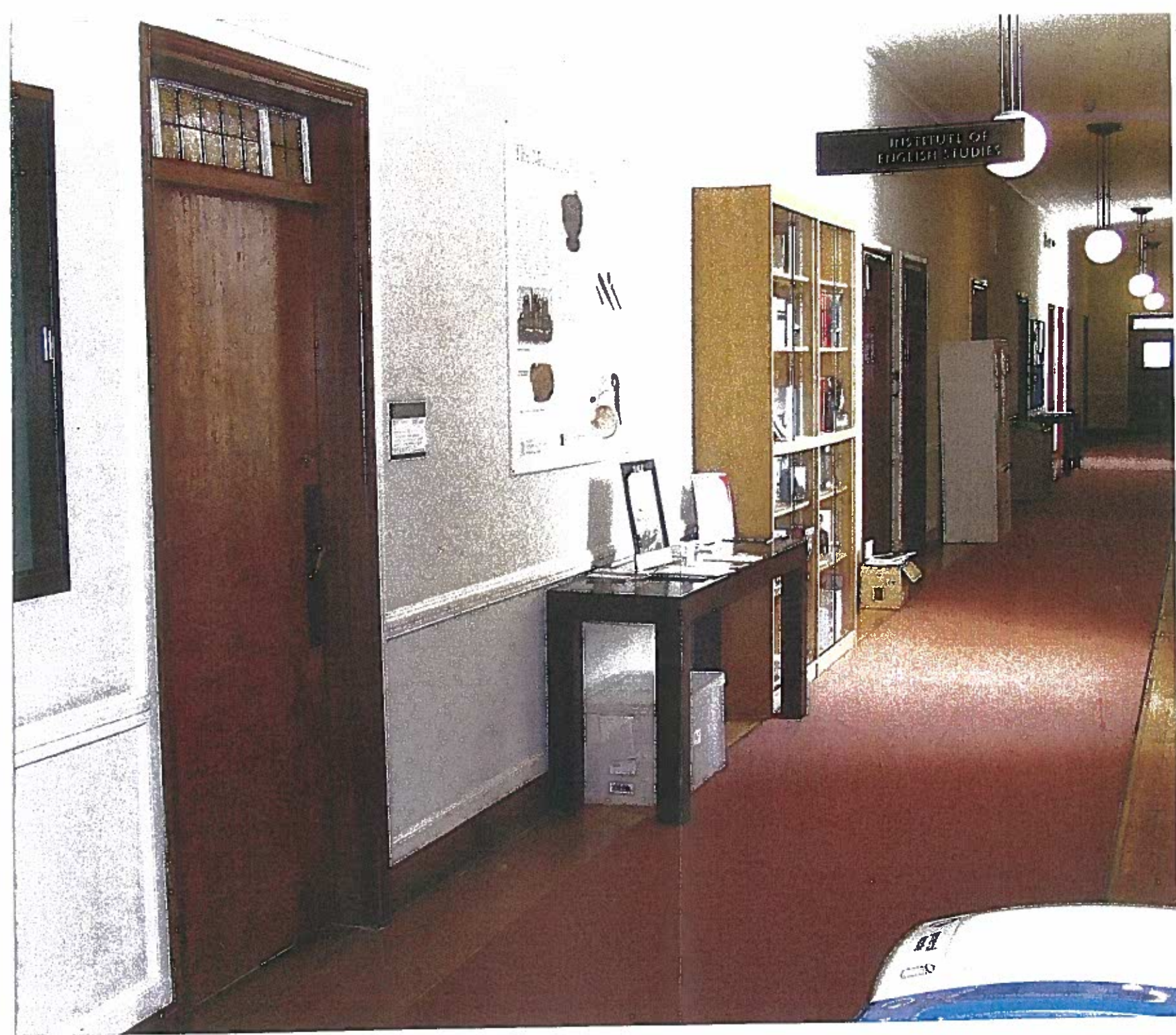
↖ * VIEW ALONG CORRIDOR. * DOOR TO 239 IN FOREGROUND. * PROPOSED DOOR TO 238 WILL BE WHERE THE LIGHT WOODEN CABINET STANDS
