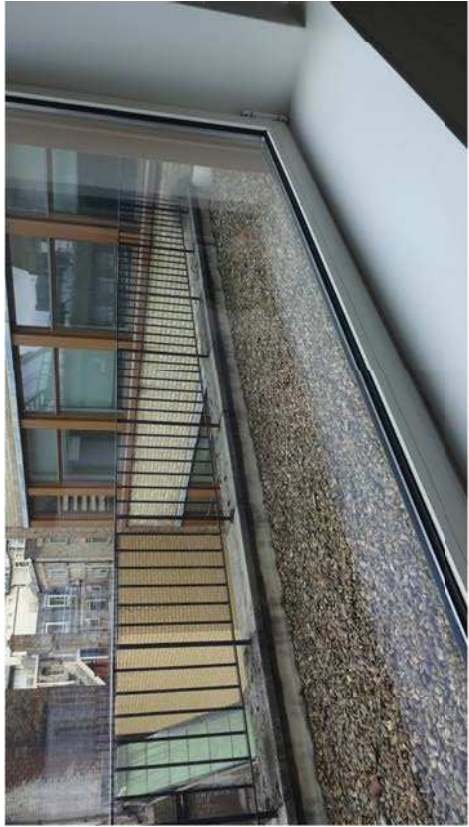
Photograph of existing non-accessible roof
