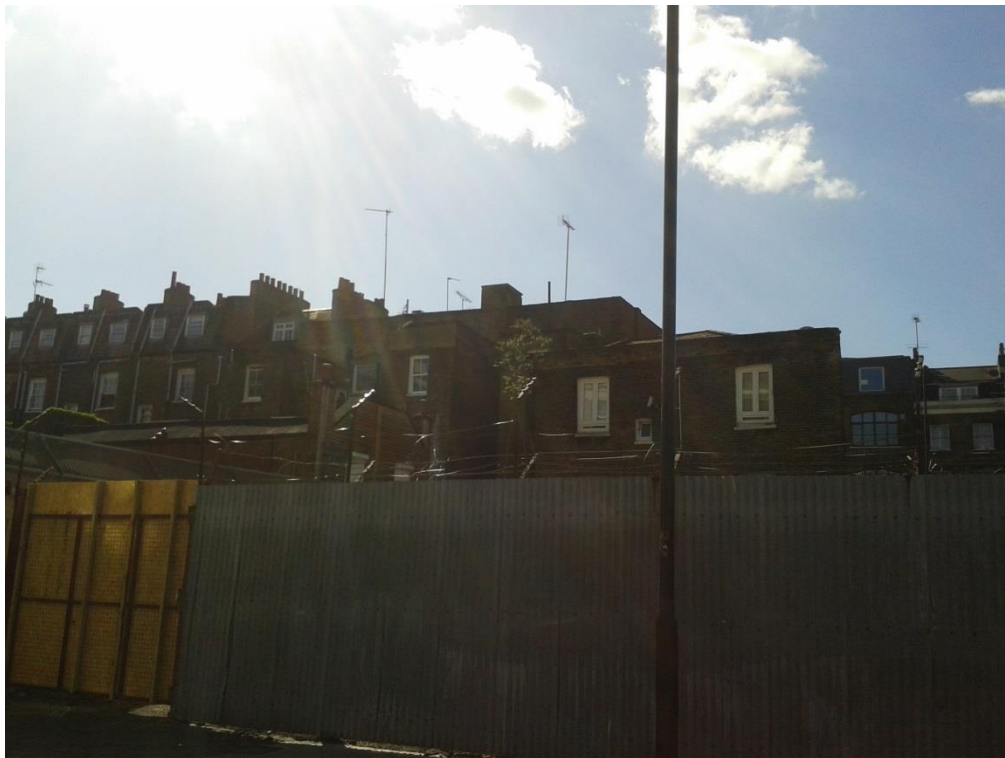
View from rear (Wicklow Street)
