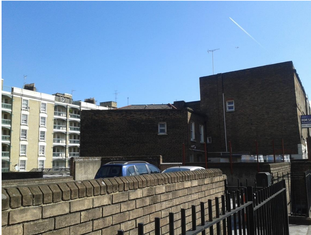
View looking east (view of side of Nos. 32 and 34)
