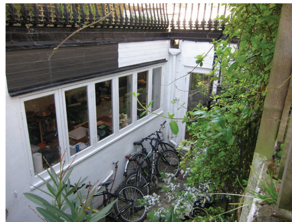
REAR KITCHEN EXTENSION AT 135 TORRIANO AVENUE WITH SMALL COURTYARD AS VIEWED BEYOND THE SCREEN
