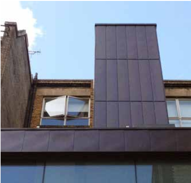
TECU Oxid metal cladding to Lewis's Building extension
