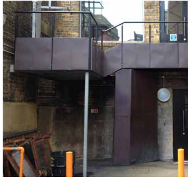
TECU Oxid metal cladding to adjoining stair case
